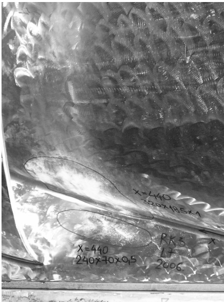
Picture 2. Cavitational damage on the back of the blade No. 7
