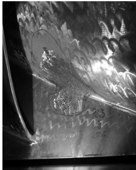
Picture 5. Cavitational damage on the back of the blade No. 3
