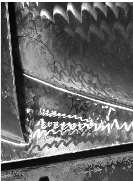
Picture 3. Cavitational damage on the back of the blade No. 13
