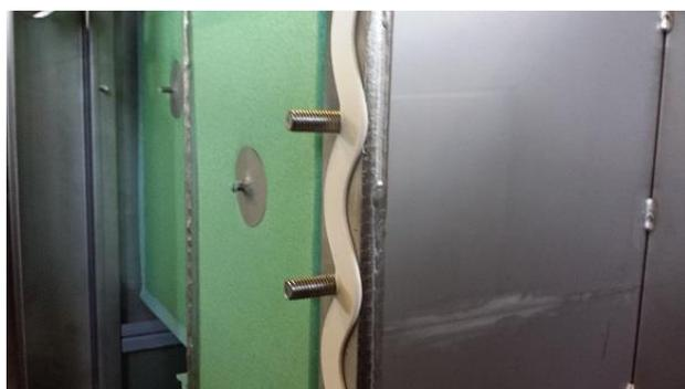
**Fig. 2.** Example of use of PTFE gaskets inside a plant for tyre moulds treatment (Courtesy Keymical)
